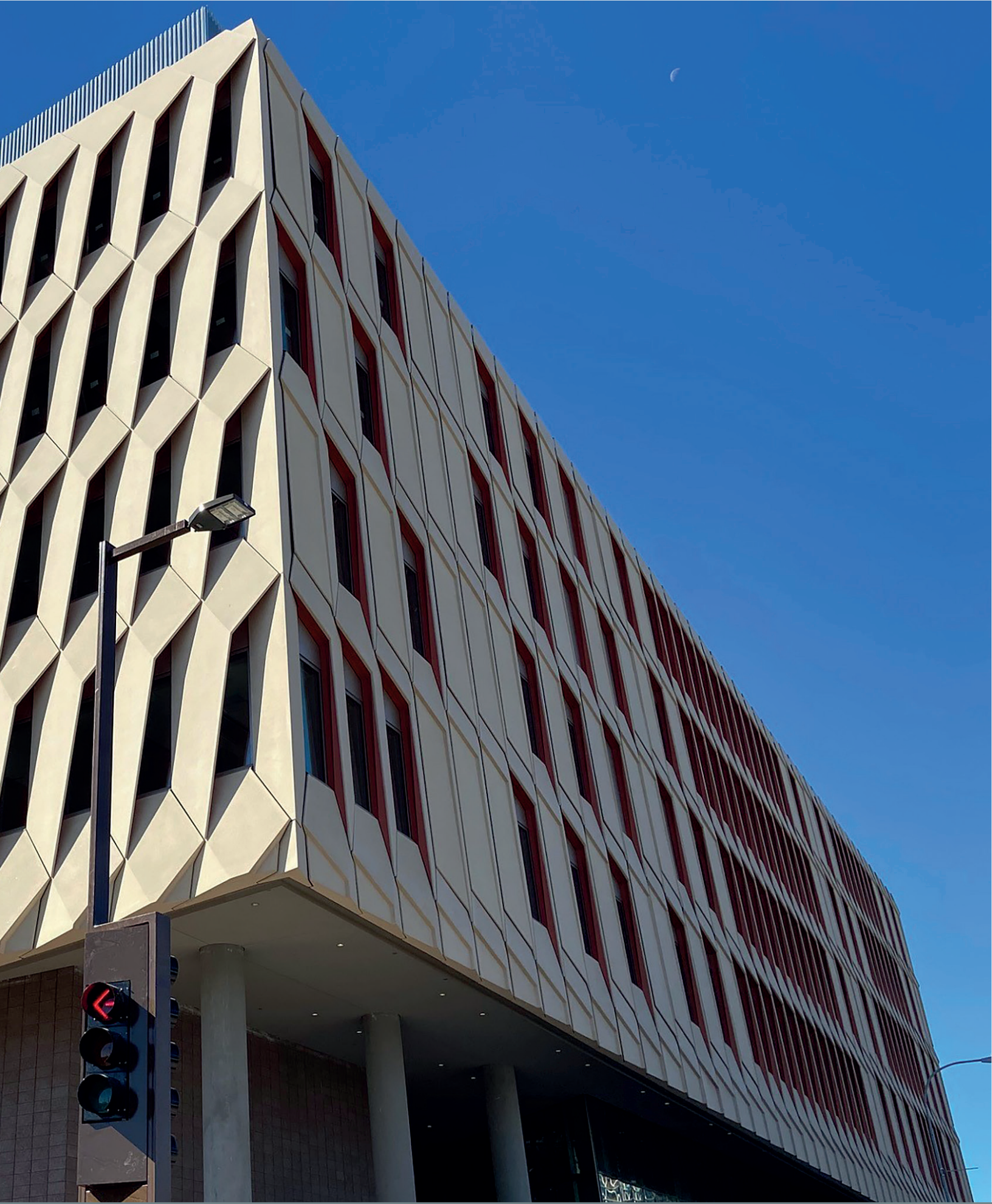
Arizona State University, ISTB-7 Building
